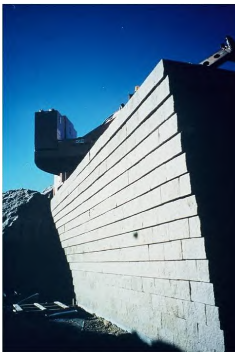
Figure 64. Photo. Negative batter wall face.
