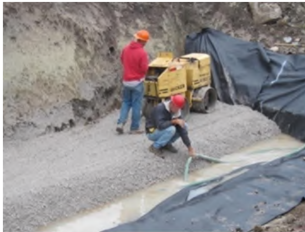
Figure 48. Photo. Dewatering during excavation of the RSF.
