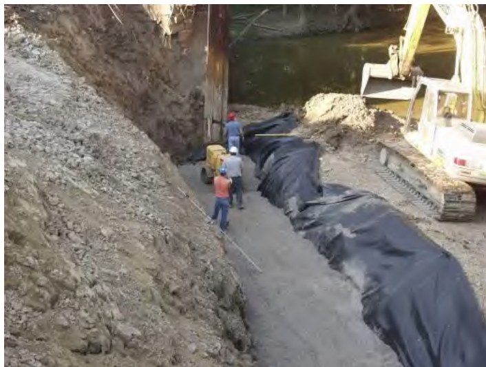
Figure 55. Photo. Encapsulation of fill in RSF.
