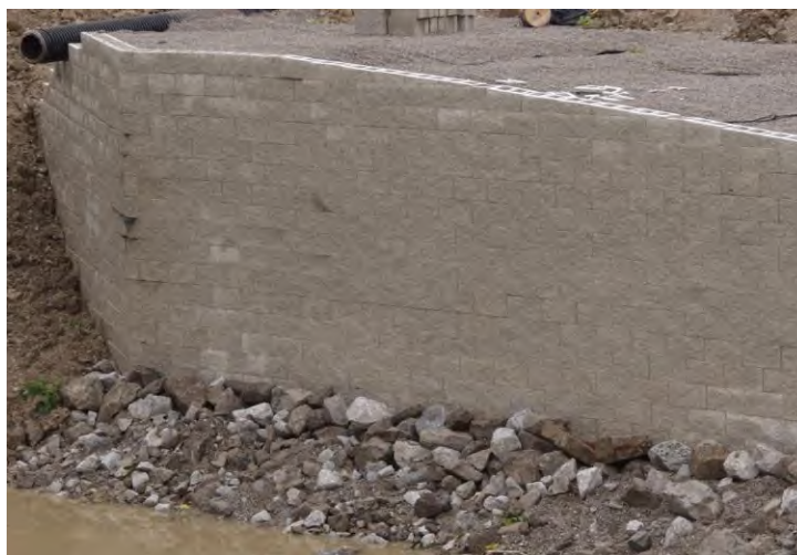
Figure 65. Photo. Blocks trimmed to match superelevation.
