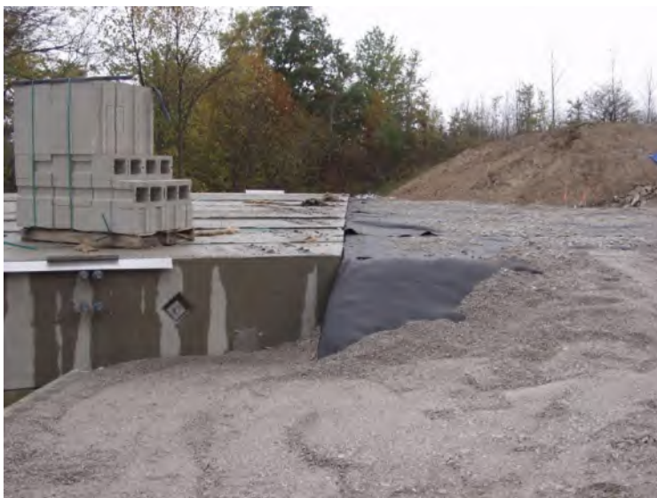
Figure 97. Photo. Completed approach fill.
