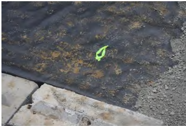
Figure 58. Photo. Completed RSF constructed within perimeter of concrete bin blocks.
