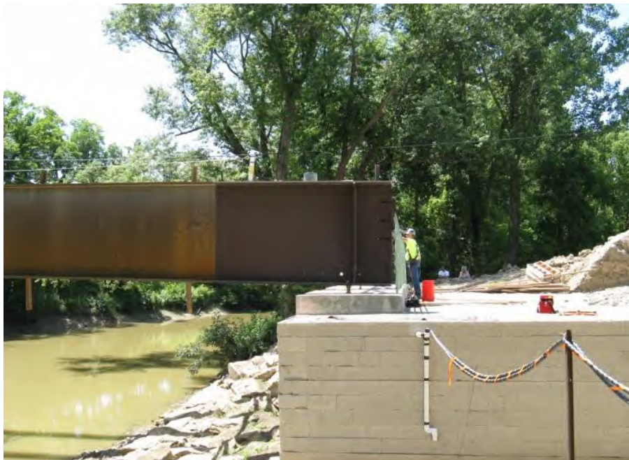
Figure 86. Photo. Steel girder on CIP footing.
