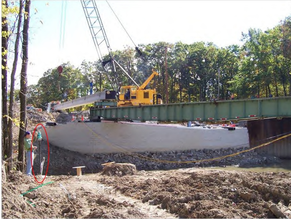
Figure 37. Photo. Location of total station reference pole.
