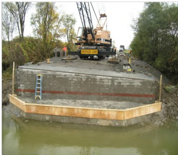
Figure 50. Photo. GRS-IBS built behind an existing concrete abutment.
