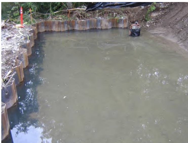
Figure 49. Photo. Sheet-pile supported excavation.
