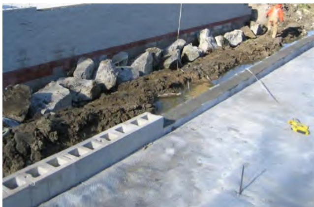
Figure 79. Photo. Bearing area block grouted prior to beam placement.
