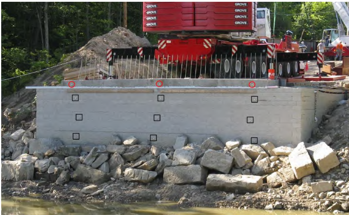
Figure 38. Photo. Location of survey targets on Tiffin River Bridge in Defiance County, OH.
