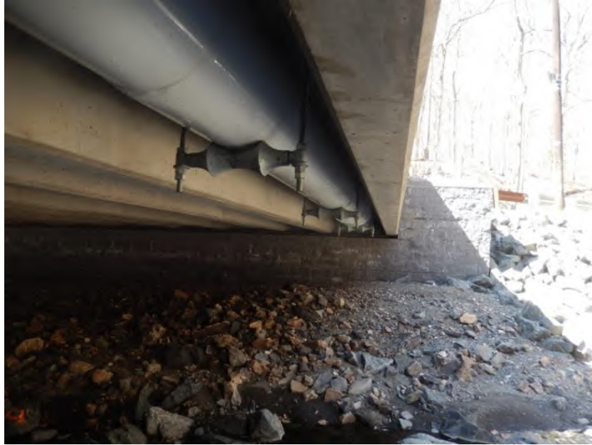
Figure 100. Photo. Utilities through a GRS abutment.
