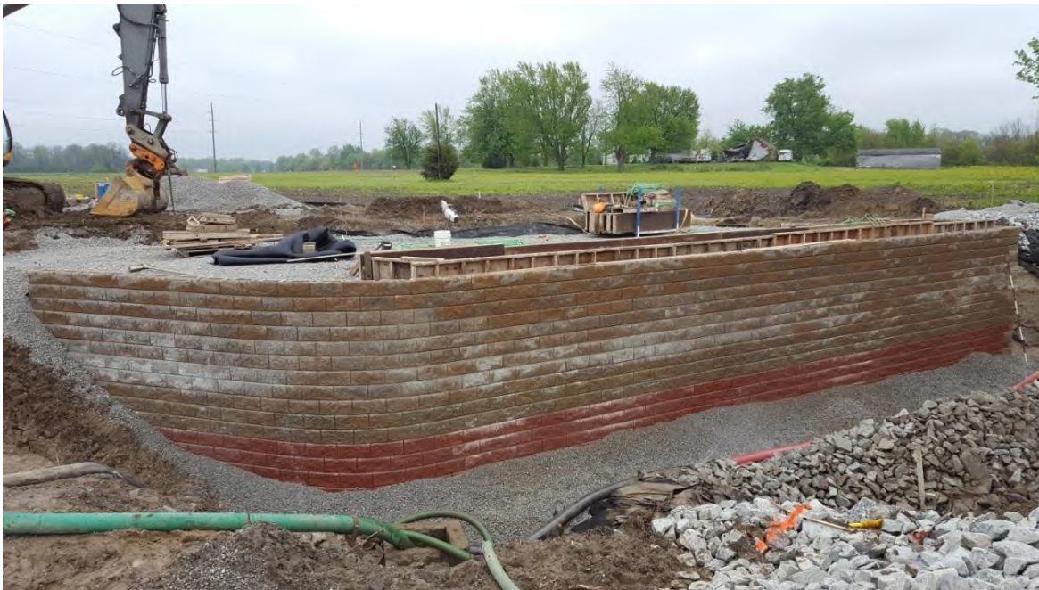
Figure 73. Photo. GRS-IBS with curved corner details under construction.
