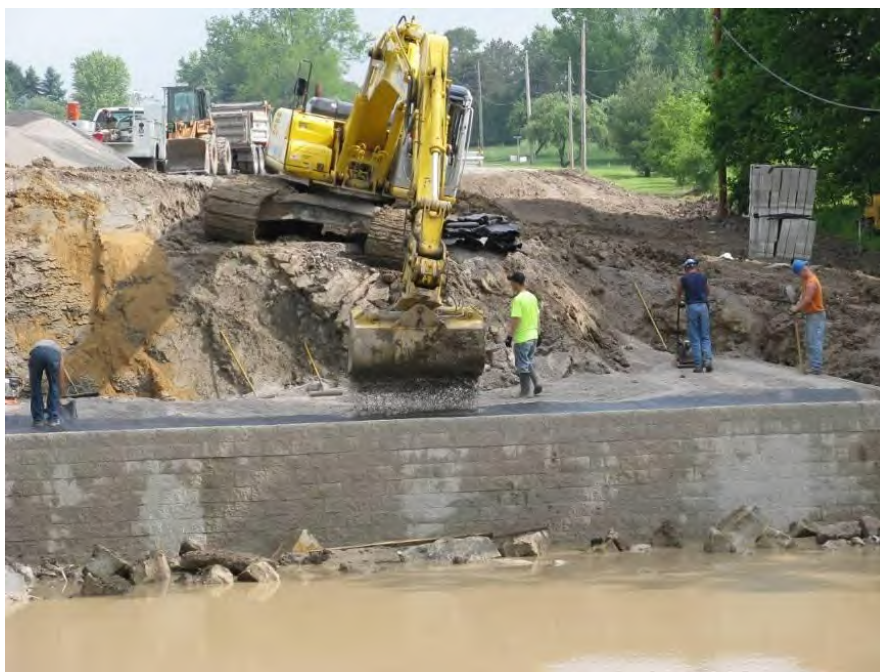
Figure 45. Photo. Typical labor crew with centrally located track hoe.
