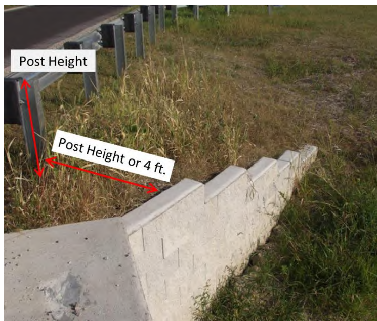
Figure 32. Photo. Guardrail lay-down distance.
