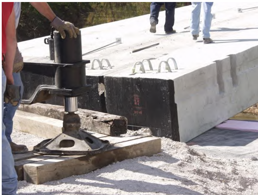
Figure 12. Photo. Bitumen coating on concrete beam ends.
