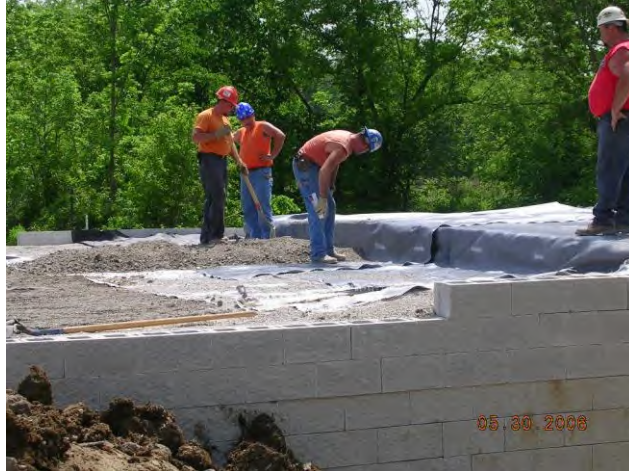
Figure 93. Photo. First 6-inch-thick fill lift.
