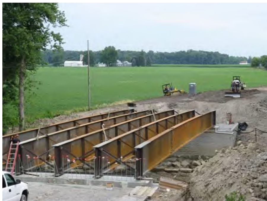
Figure 86. Photo. Steel girder on CIP footing.
