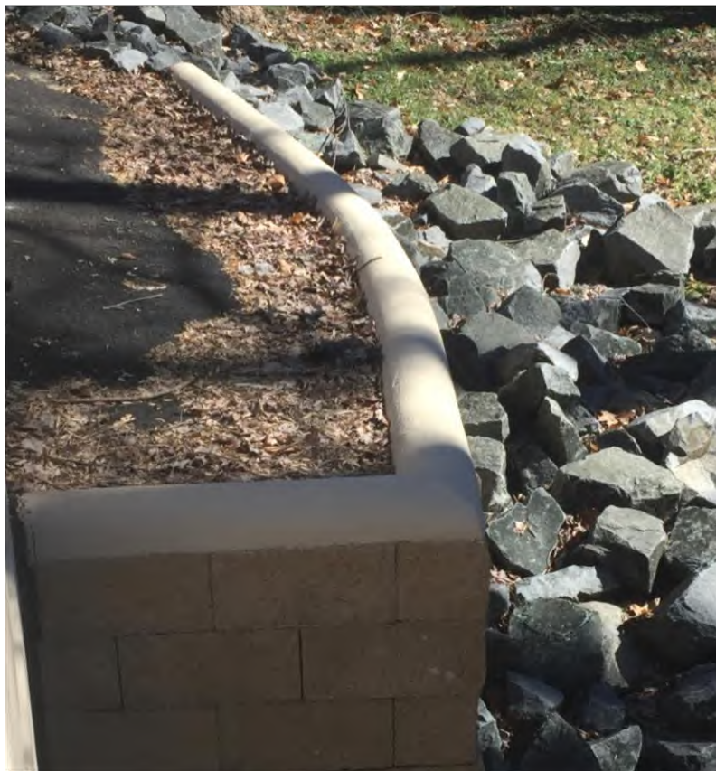
Figure 71. Photo. Alternative wing wall acute angle corner detail with CMU blocks.
