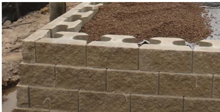
Figure 10. Photo. GRS abutment constructed with an SRW block facing.
