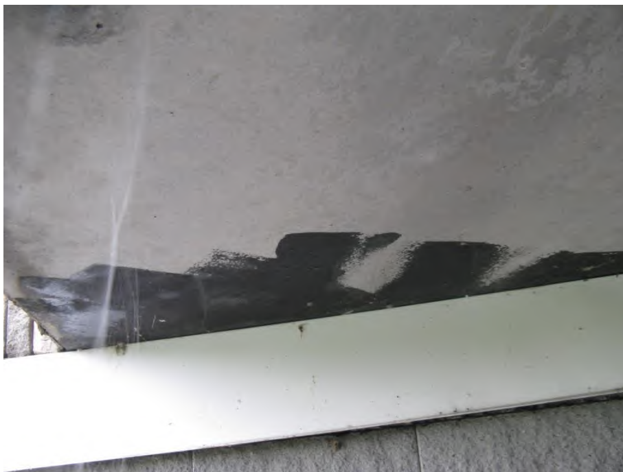
Figure 13. Photo. Bitumen coating under voided slab beam.
